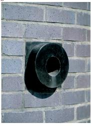
The outlet of the rainwater pipe from the monostyle column was cast in black concrete and then clear-lacquered to shine a deep sable.
