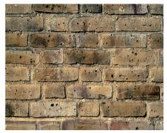
Old brickwork laid in lime mortar has small pieces of grit in its wide joints. There is none of the dead grey of Portland cement. The depth of the mortar joint is gentle - outlining the separate bricks while preserving the wholeness of the wall as a great sheet.
