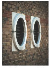
Ventilation extracts. Nothing was allowed to penetrate the masonry skin unless it was fortified by a massive and solid cast ballidon limestone grommet.
