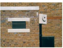
When unavoidably interior to the walls, JOA gutters are always fitted with prominent overflow outlets. This was a rainwater hopper, and overflow, in ballidon limestone concrete, to the transformer building.
