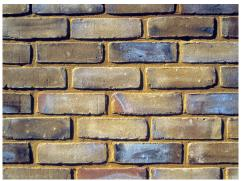
In Kensal Road the mortar was 'pointed' by being scraped back 5 mm with an American hand-held wheeled trowel. Some suppose this endangers bricks to frost attack - again betraying an ignorance of how stock bricks resist freezing. The effect is purely aesthetic.
