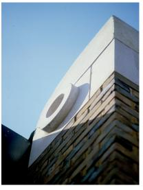
Corner 'acroteria' doubling as ancient horn-images, gutter overflows and brick wall compressors.
