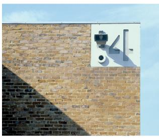
This, marking-out the Unit - bays at Poyle, was the first of the many 'capitals' invented by JOA. Its body, that is to say the column below it, was securely buried in the brick walls beneath. The odd numbers had the light and gutter overflow composed as an exclamation mark. It was made by casting white onto grey concrete and then removing polystyrene shapes to give the stencil-font digit.
